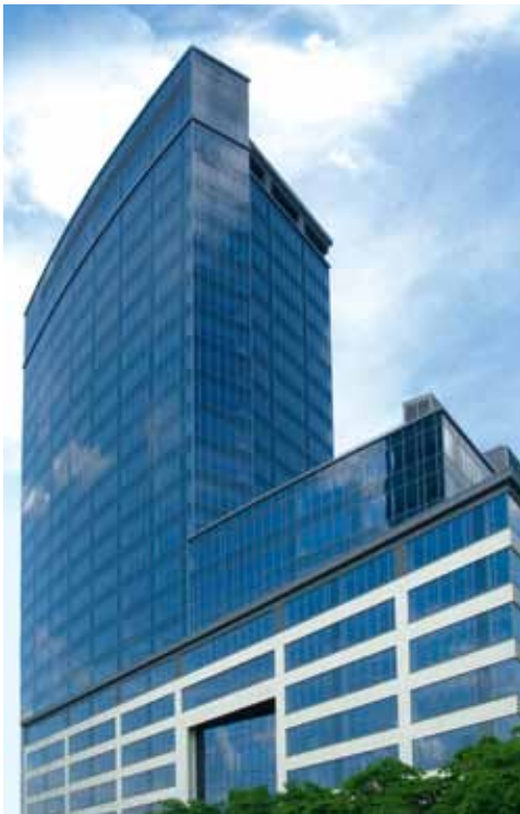
BELVEDERE CENTRE (NORTH GATE), Warsaw, Poland
