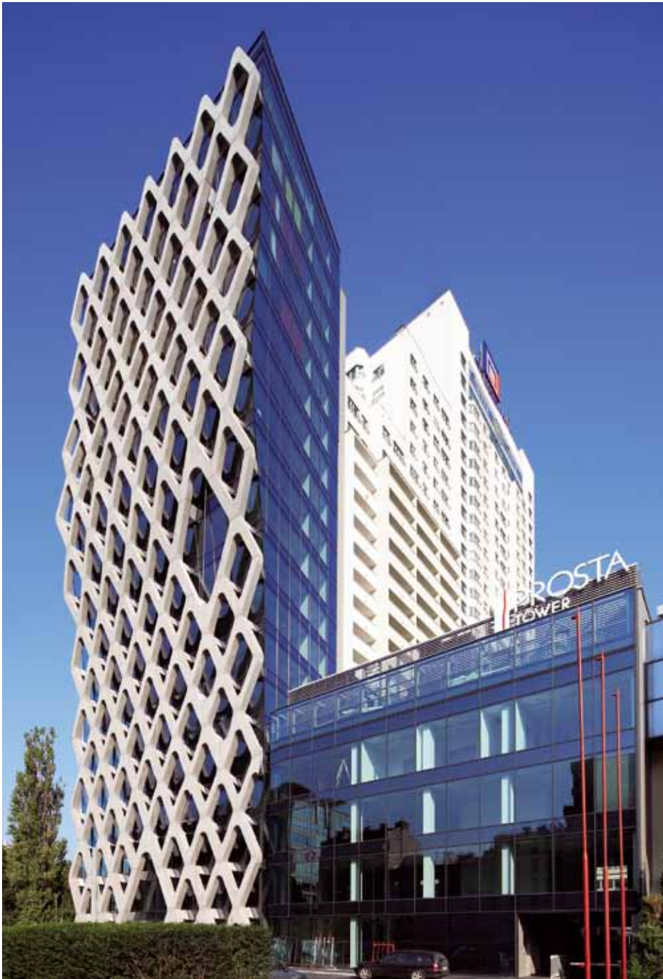
PROSTA TOWER, Warsaw, Poland
